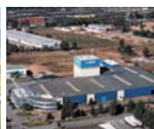
Mapei France S.A. Saint Alban (Toulouse) France
