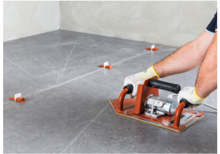
Tapping the tile by hand or going over the surface with a vibro-plate
