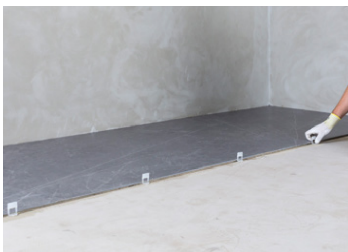
Placing the spacers in position
