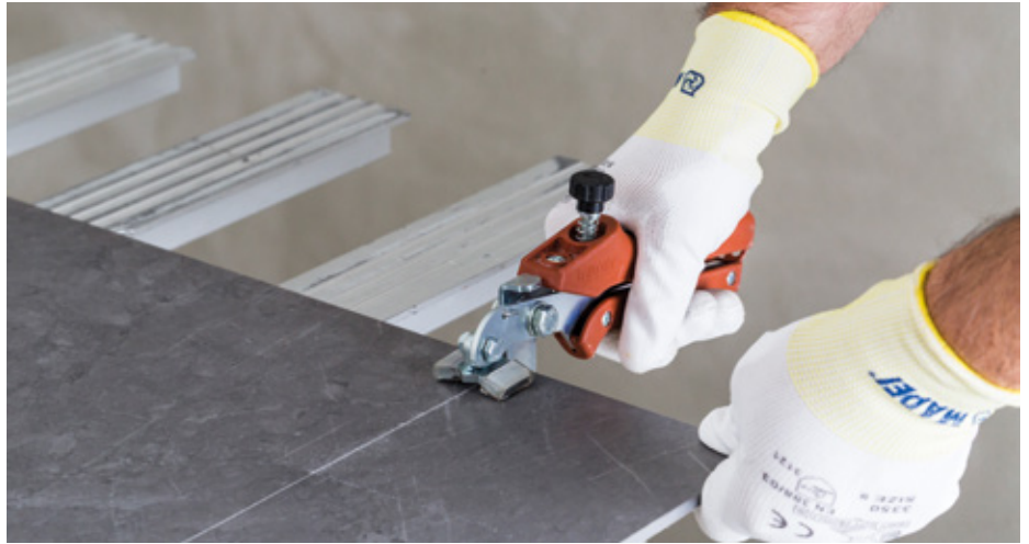
Creating a fracture with tile snips
