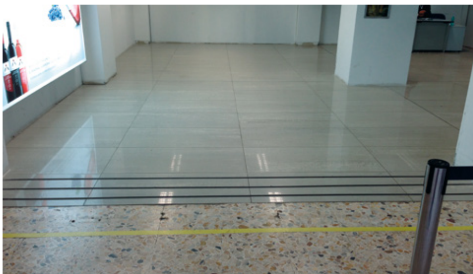
Installing tiles over an old floor
