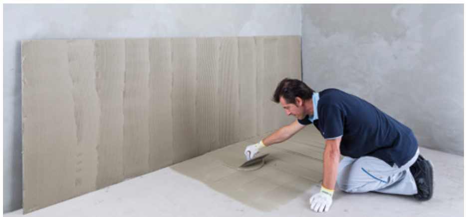
Installing a tile using the double-buttering technique
