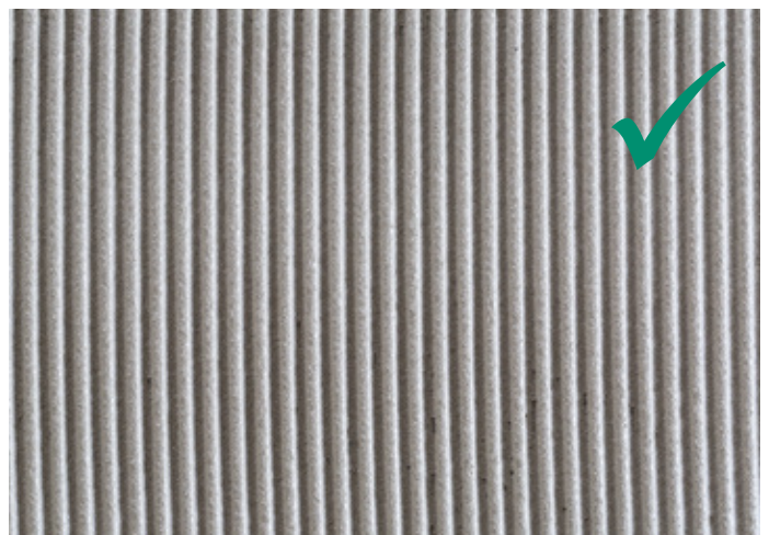
How to spread the adhesive correctly
