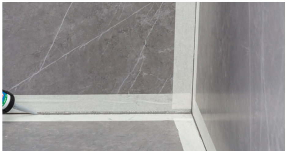
Perimeter joint sealed with MAPESIL AC
