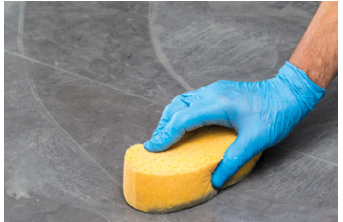
Cleaning the grout with a Scotch-Brite pad finishing off the grouted tiles with a sponge
