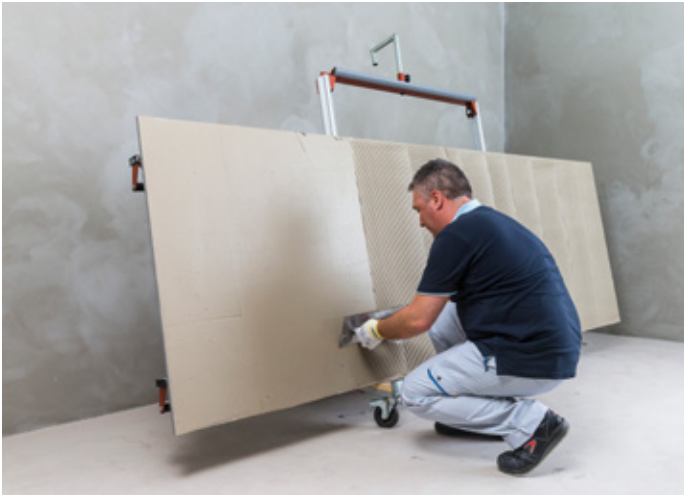
The adhesive is spread in the same direction on the back of the tile and on the substrate
