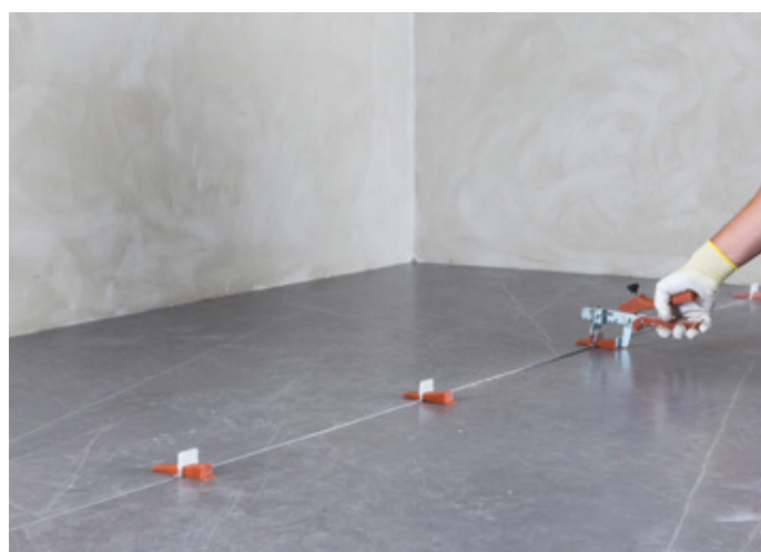
Placing the spacers in position
