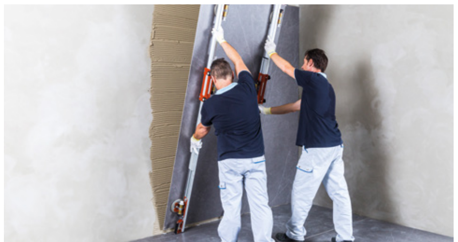
Installing a wall tile
