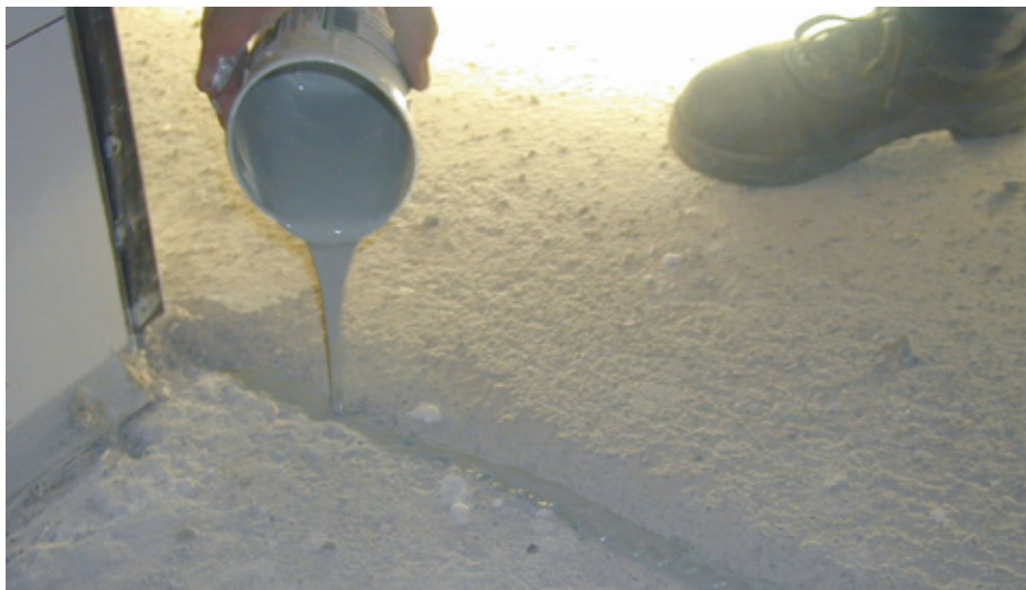
Sealing cracks in a substrate with EPORIP
