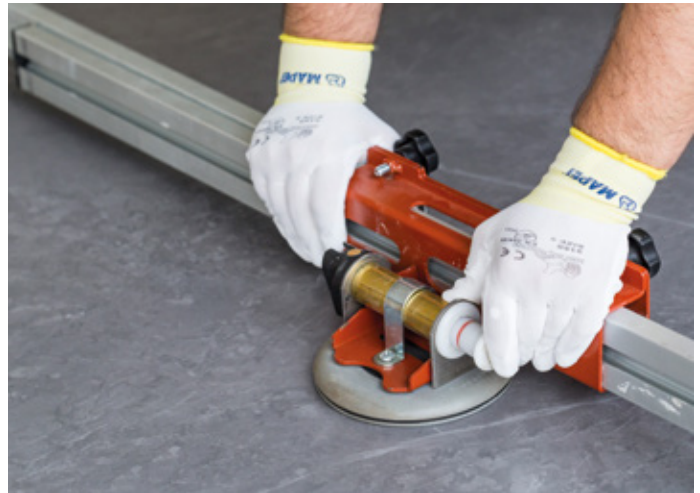
Applying a pump-action suction cup
