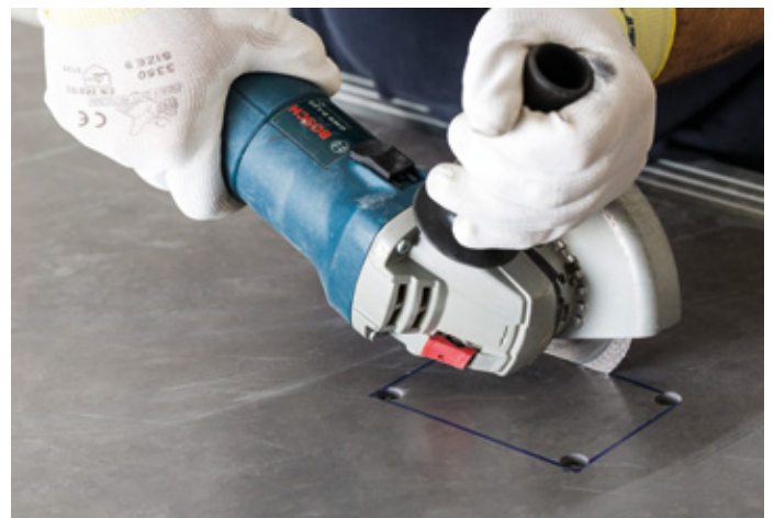
Sequence to make a rectangular hole
