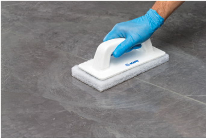
Cleaning the grout with a Scotch-Brite pad finishing off the grouted tiles with a sponge
