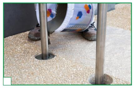
When mixed with water, **Mapegrout Anchor & Repair** forms hi-flow mortar applied in a single layer at a thickness of 5 cm, after having prepared the substrate.
