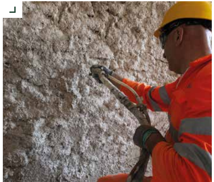
Application of PLANITOP INTONACO ARMATO by spray
