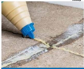
TWO-COMPONENT SILICATE-URETHANE RESIN
