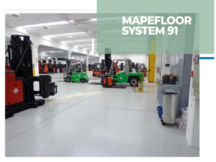
Trowelled epoxy mortar system for industrial floors, ideal for renovating old floors; thickness 6 to 15 mm.
