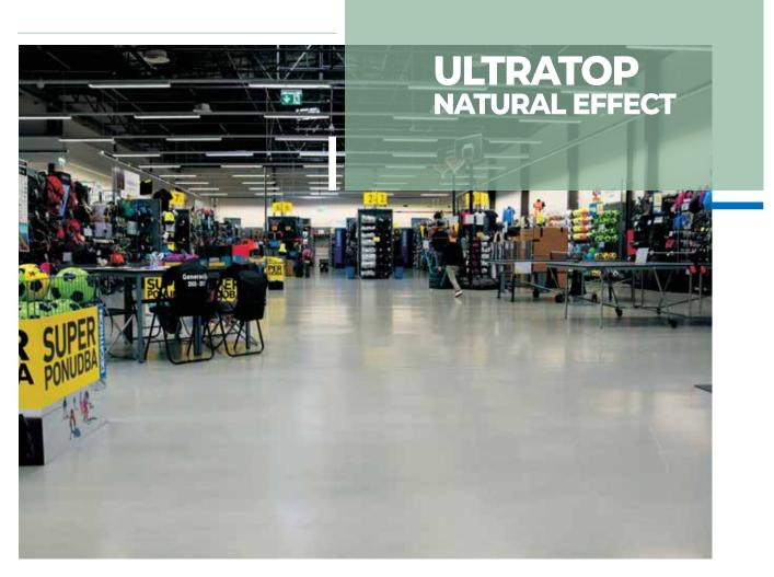
Self-levelling, ultra-fast setting cementitious system for abrasion-resistant floors; thickness 5 to 40 mm.
