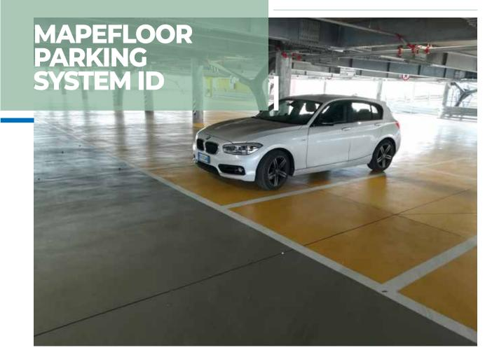
Multi-layered, seamless polyurethane system with good dynamic crack-bridging capacity for pedestrian surfaces and areas with vehicle access exposed to intense traffic indoor. The system complies with Rili DafStb (Guideline of the German Committee on Reinforced Concrete) OS 13 and the concrete surface protection systems according to EN 1504-2. Total thickness 2 to 2.5 mm.
