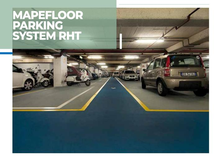
Multi-layered, seamless epoxy system for pedestrian areas and surfaces with vehicle access exposed to intense traffic. The system complies with Rili DafStb (Guidelines of the German Committee on Reinforced Concrete) OS 8 and the concrete surface protection systems according to EN 1504-2; thickness 3 to 3.5 mm.
