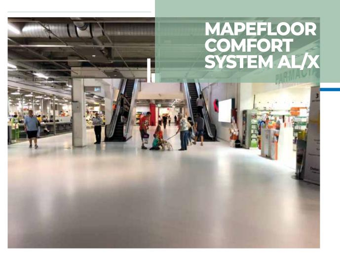
Self-levelling, elastic, flexible, aliphatic polyurethane resin-based system resistant to UV rays for coating surfaces in civil surroundings; thickness 6 mm.
