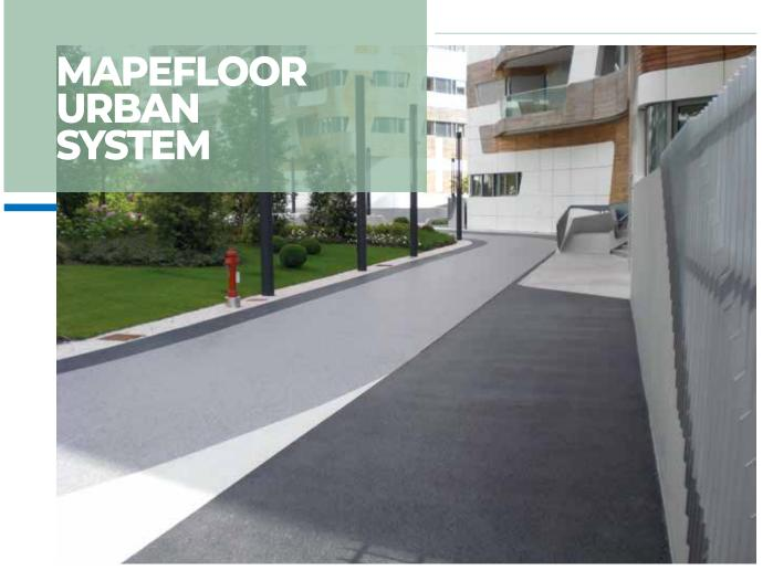
Self-draining system based on aliphatic polyurethane-based binder mixed with natural aggregates (2-4 mm or 4-8 mm) for creating decorative external surfaces.
