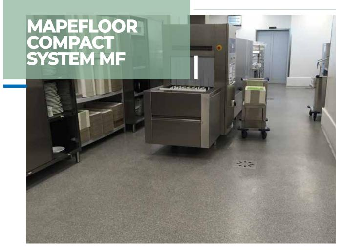
Multi-layered decorative epoxy system with a highly attractive finish for industrial and commercial floors; thickness 2.5 to 3.0 mm.
