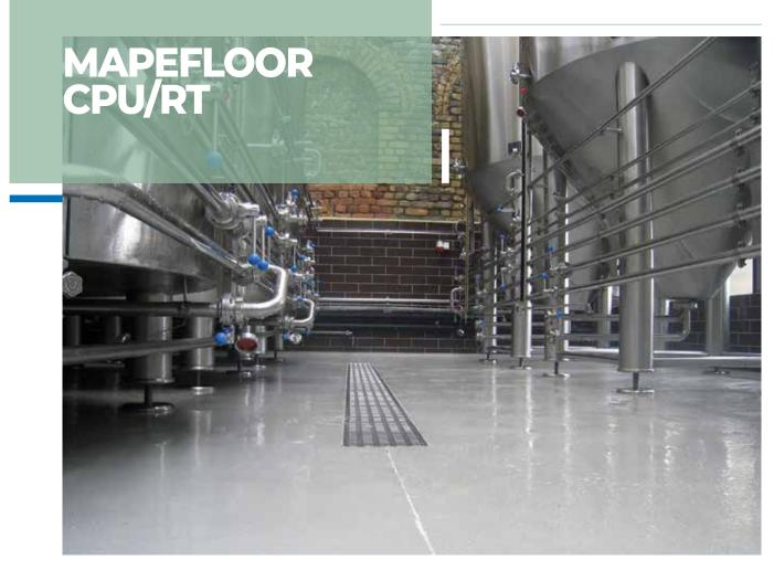
Easy-to-apply, high-strength, polyurethane/cement-based mortar system with high mechanical strength, resistance to chemicals and thermal shock for antiskid coating of industrial floors; thickness 6 to 9 mm.
