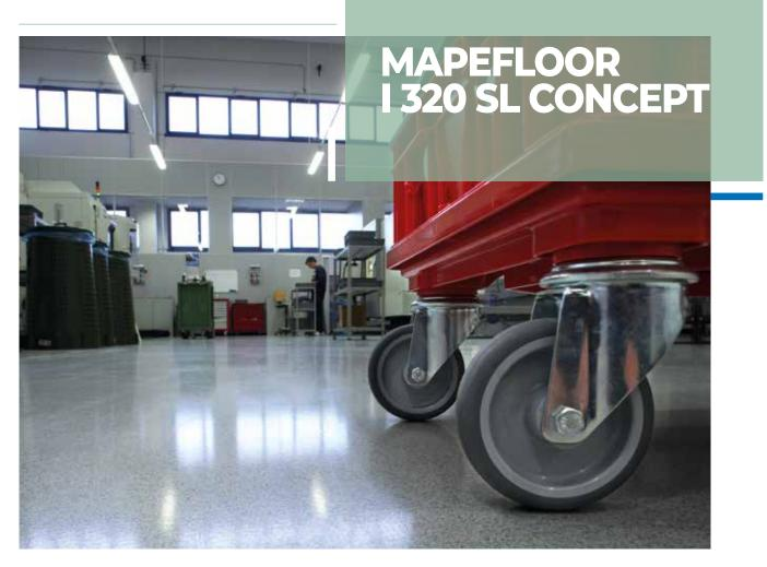
Self-levelling epoxy system with a coloured granular finish for decorative floors; thickness of approx. 2 mm.
