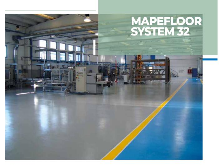
Multi-layered epoxy system with high solids content for industrial floors; thickness 3 to 3.5 mm.
