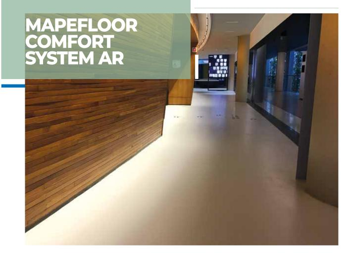
Self-levelling, elastic, aromatic polyurethane resin-based system resistant to UV rays for coating surfaces in internal surroundings; thickness 2 mm.
