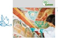
Super-fluid, salt-resistant, fillerized hydraulic binder, based on lime and Eco-Pozzolan, for making injection slurries for consolidating masonry and render, including the frescoed one
