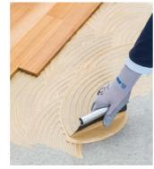
APPLICATION n. 2 or 4 notched trowel for wood CONSUMPTION 1.0-1.5 kg/m<sup>2</sup> COLOUR comp. A: beige or brown; comp. B: whitish PACKAGING 10 kg drums (A+B)
