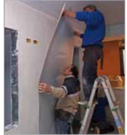
Fig. 4.5 - Installing a wall covering where adhesive with high initial hold is required
