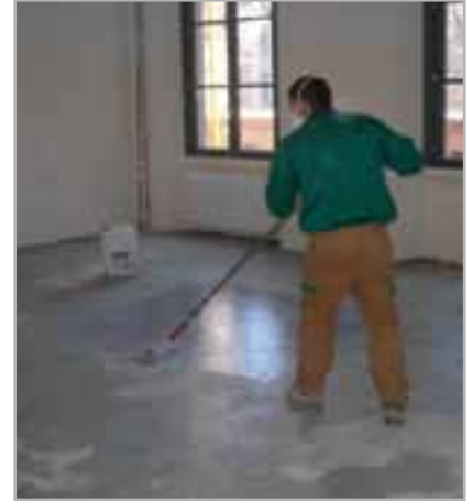
Fig. 5.1 - Application of adhesion promoting primer
