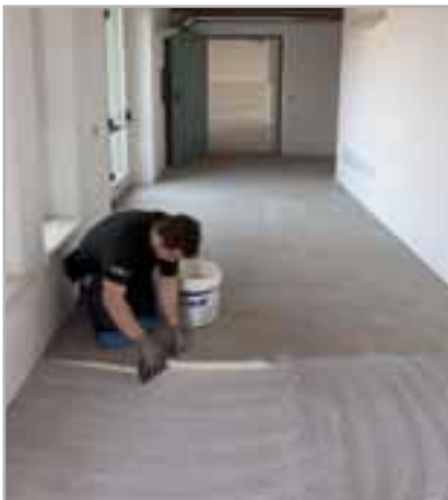
Fig. 5.5 - Application of adhesive with a suitable notched trowel
