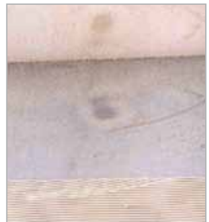
Fig. 5.9 - Emptying the adhesive from under floor covering
