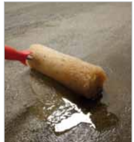
Fig. 5.2 - Application of consolidating/waterproofing membrane
