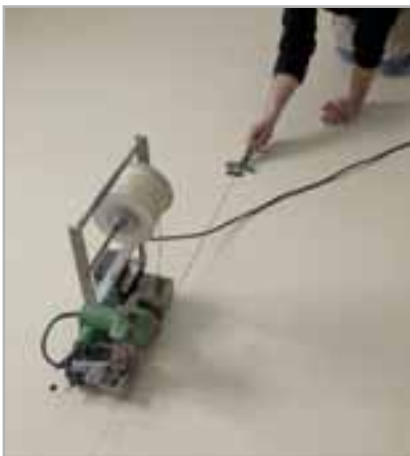
Fig. 4.15 - Sealing rubber flooring
