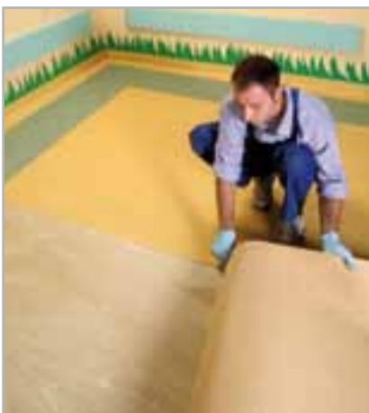
Fig. 5.6 - Installation of covering in sheet form on adhesive with sufficient tack
