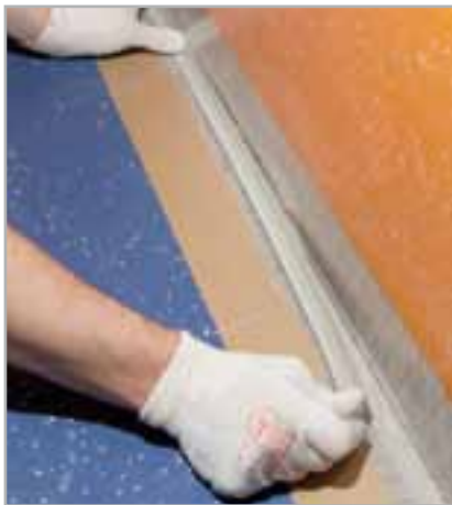
Fig. 5.11 - Application procedure for fillets using MAPECONTACT
