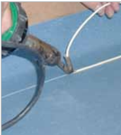
Fig. 4.14 - Sealing rubber flooring
