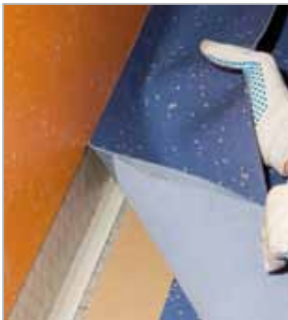
Fig. 5.12 - Application procedure for fillets using MAPECONTACT
