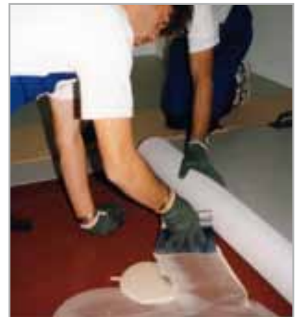
Fig. 3.8 - Installing PVC flooring over MAPELAY using ADESILEX G20
