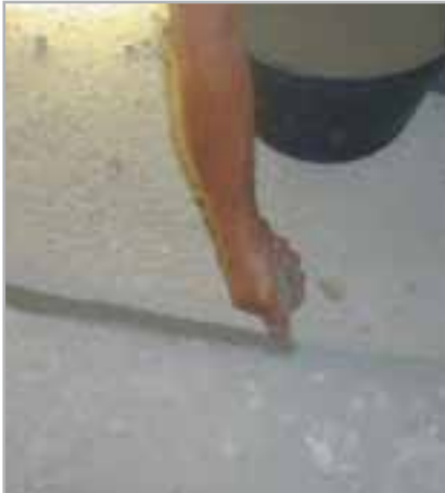
Fig. 3.10 - Sand blinding on the surface of fresh EPORIP
