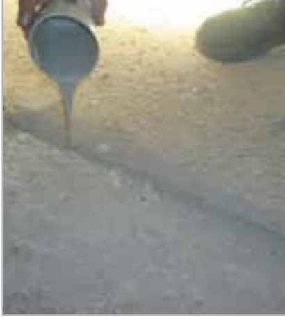
Fig. 3.9 - Sealing a cracked screed by applying EPORIP
