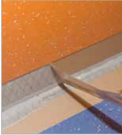
Fig. 5.10 - Application procedure for fillets using MAPECONTACT
