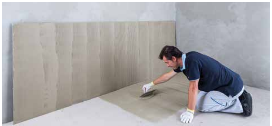
Installing a tile using the double-buttering technique
