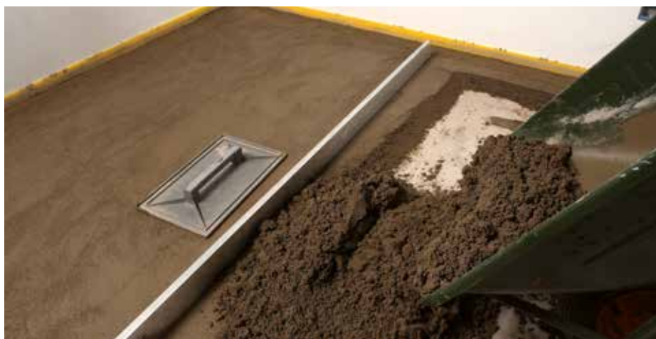
Installing a screed made from TOPCEM PRONTO
