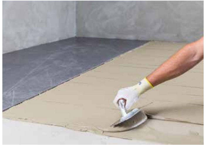
The adhesive is spread in the same direction on the back of the tile and on the substrate
