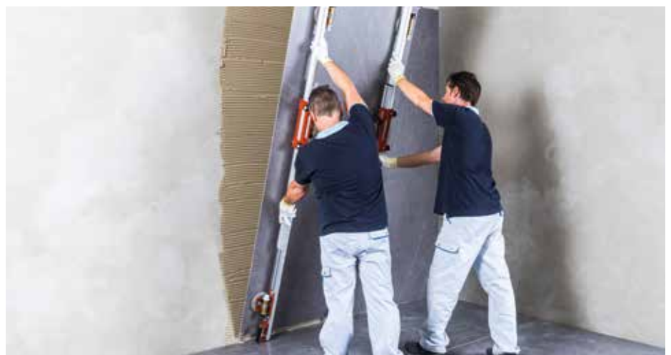
Installing a wall tile
