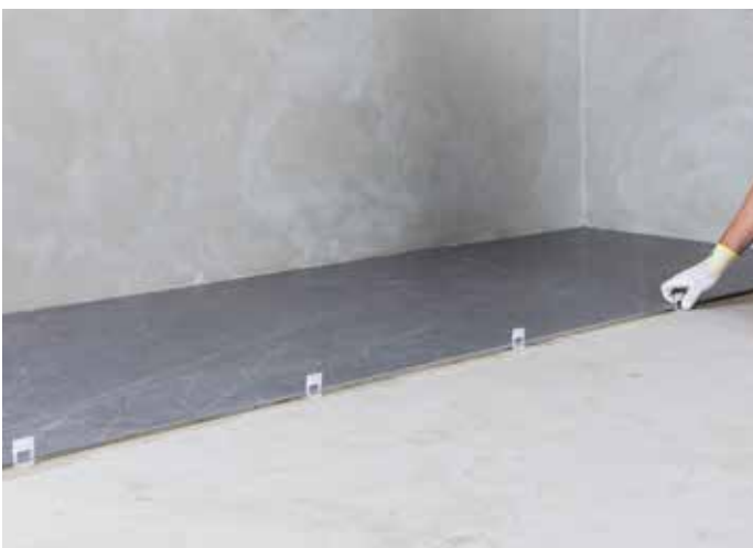
Placing the spacers in position
