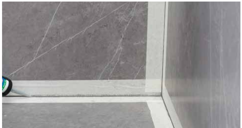
Perimeter joint sealed with MAPESIL AC
