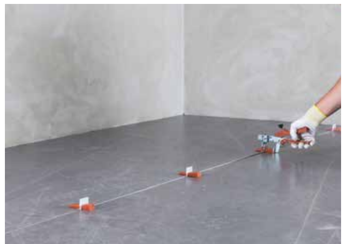
Placing the spacers in position
