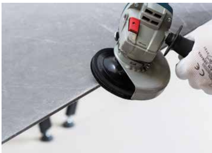
Smoothing off the cut edges
