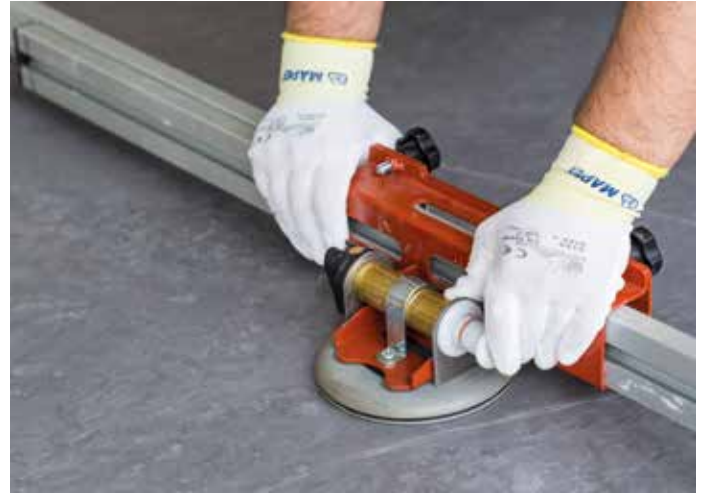
Applying a pump-action suction cup
