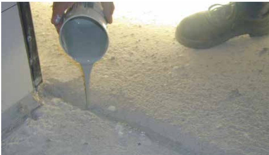
Sealing cracks in a substrate with EPORIP
