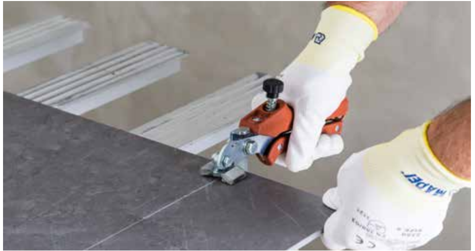
Creating a fracture with tile snips
