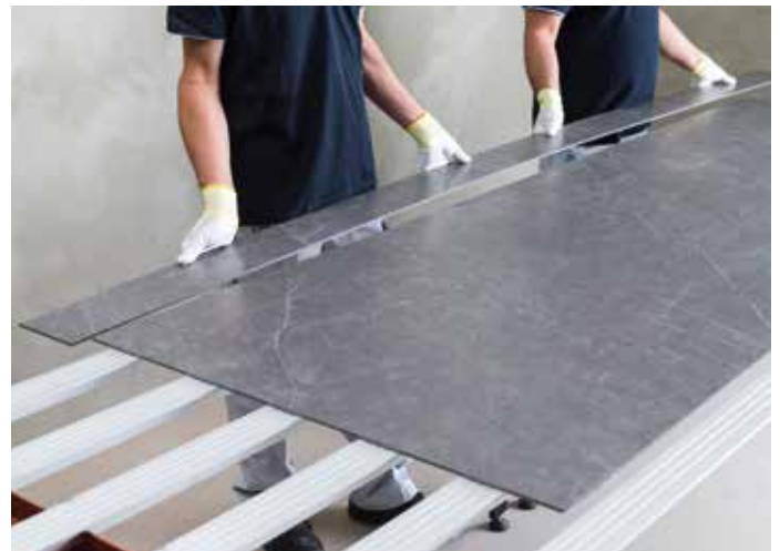
Breaking the tile in two
