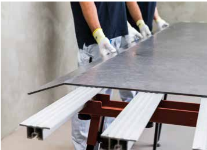
Breaking the tile in two
