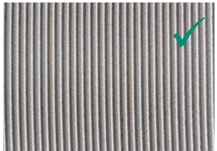
How to spread the adhesive correctly
