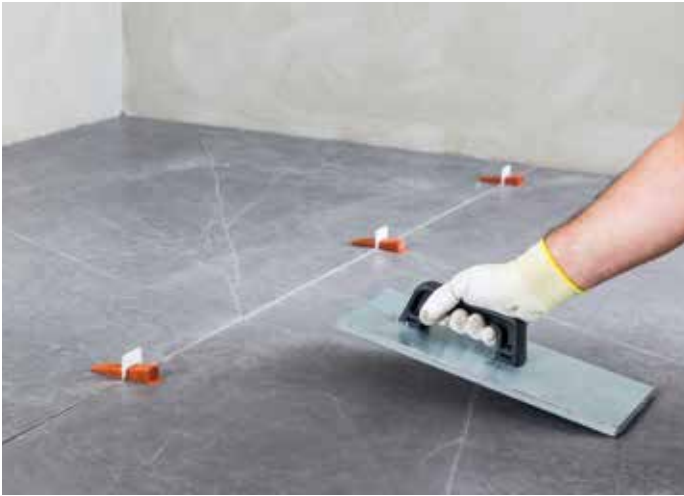
Tapping the tile by hand or going over the surface with a vibro-plate
