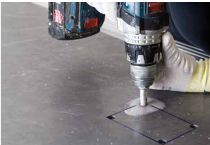
Sequence to make a rectangular hole
