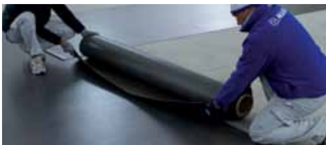
Rolling out the fibre-reinforced PVC mat
