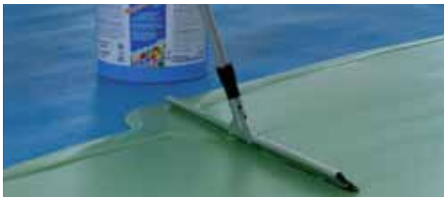
Applying the acrylic coloured coating Mapecoat TNS Finish
