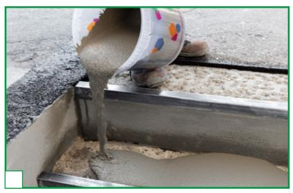
Fibre-reinforced, compensated-shrinkage mortar for repairing concrete and anchoring metal structures by pouring the mortar into specially prepared areas.
