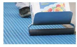
Go over the membrane with a float or roller and press it down (maximum 35 kg).
