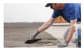
Spread the adhesive over the surface of the substrate with a 5 mm notches trowel.
