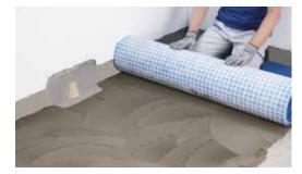
Lay **Mapeguard UM 35** membrane over the adhesive while it is still wet.
