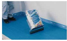
Go over the membrane with a float or roller and press it down (maximum 35 kg).
