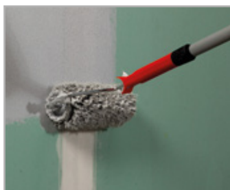
Spreading the first coat of MAPEGUM WPS
