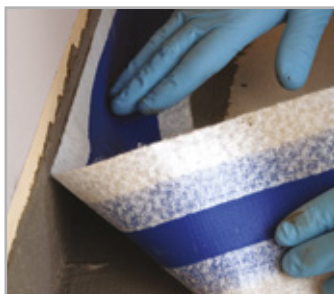
Application of MAPEBAND with MAPELASTIC SMART
