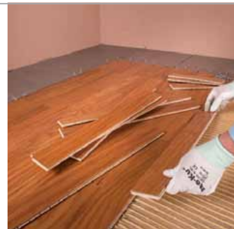
Fig. 5.7 - Spread the adhesive to bond parquet
