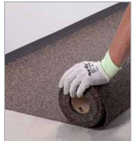
Fig. 5.4 - Unroll the sheets of MAPESONIC CR
