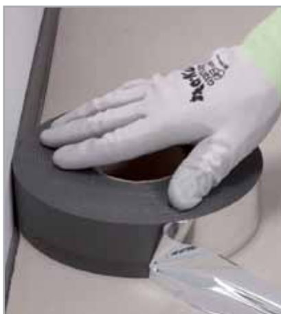
Fig. 5.2 - Apply MAPESONIC STRIP around the perimeter
