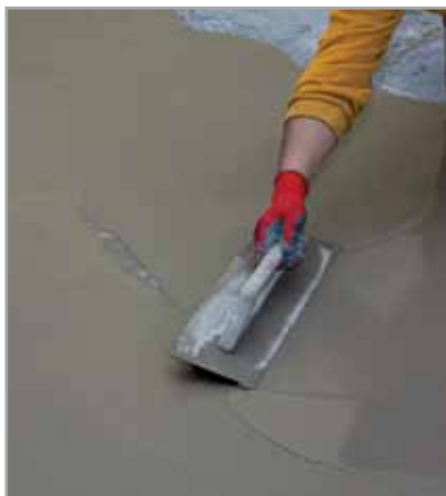
Fig. 5.1 - Levelling of the substrate
