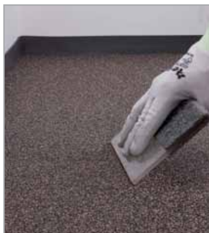
Fig. 5.5 - Massage the surface of MAPESONIC CR
