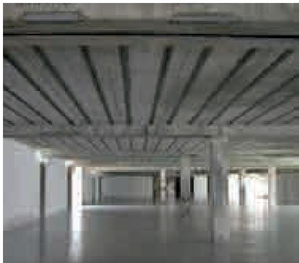
Flexural strengthening of beams and a floor with CARBOPLATE SYSTEM
