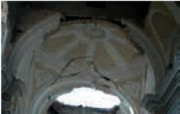
Collapse of masonry vaults
