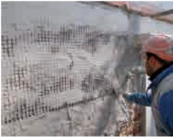
**Application of a compact strengthening package to increase the shear-tensile strength of bay walls**
