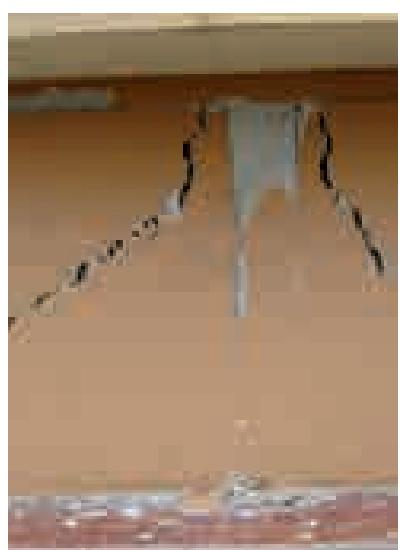
Shear failure of partition walls
