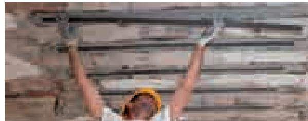
Application of CARBOPLATE SYSTEM on crack-cement floor joists
