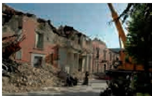
Masonry with poor mechanical properties
