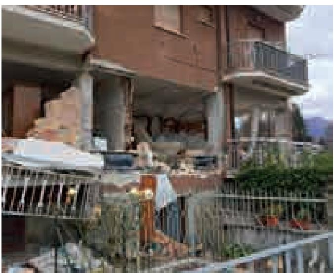
Collapse of external buffer walls
