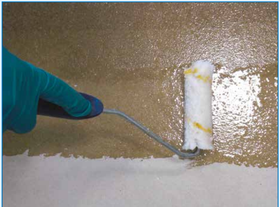
Application of Mapefloor I 910 as adhesion promoter
