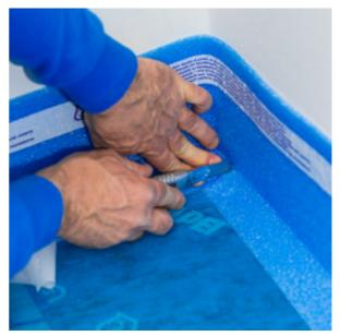
At the corners, cut the lower horizontal part of **Mapesilent Band R** where necessary
