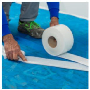
After checking that the sheets of **Mapesilent Roll** overlap perfectly, seal all overlaps using **Mapesilent Tape**
