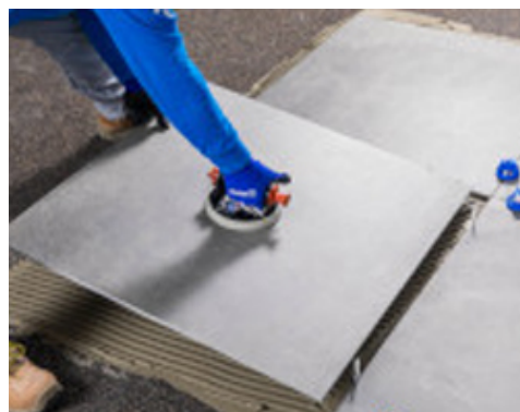
Spread the adhesive on Mapesonic CR and bond the new floor finish
