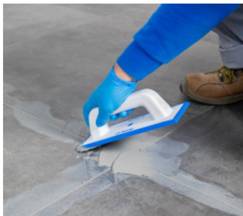
Grout the surface of the room
