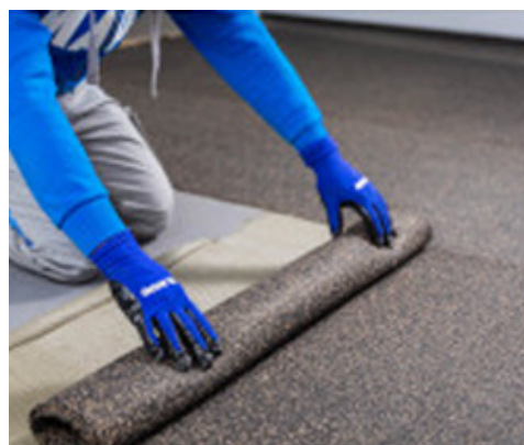
Unroll the sheets of Mapesonic CR on the surfaces to be soundproofed
