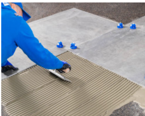
After suitable preparation of the substrate, spread on the adhesive to bond the soundproofing sheets
