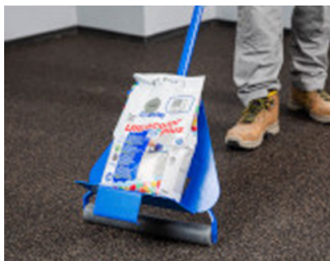
Massage the surface with a rigid roller or flat trowel, starting from the centre and working towards the edge
