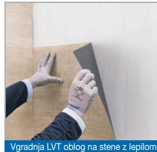
Vgradnja LVT oblog na stene z lepilom Ultrabond Eco MS 4 LVT Wall.
