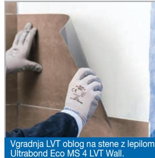
Vgradnja LVT oblog na stene z lepilom Ultrabond Eco MS 4 LVT Wall.
