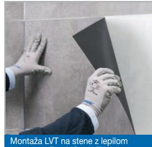
Montaža LVT na stene z lepilom Ultrabond Eco MS 4 LVT Wall.
