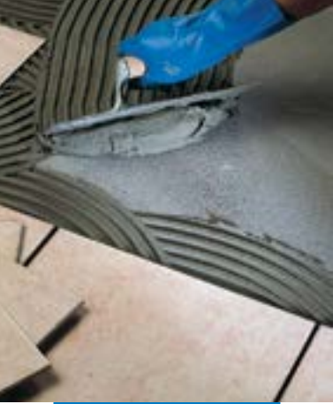
Installation of single-fired tile on floor
