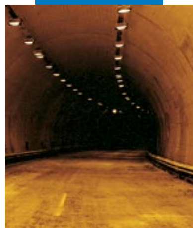
Application of Planiseal 88 by spray gun in highway tunnel
