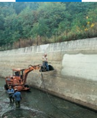
Application of Planiseal 88 by spray gun in hydroelectric canal
