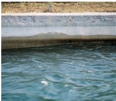
hydroelectric canal - Surfaces treated with Planiseal 88
