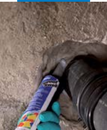
Through element sealed using Mapeproof Swell
