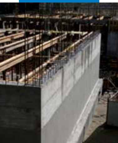
Retaining wall waterproofed after casting using Mapelastic Foundation
