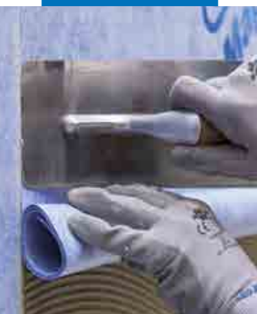
Application of the second sheet
