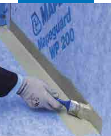
Application of the Mapeguard WP Adhesive in order to seal the joints in the corner before the application of Mapeguard ST
