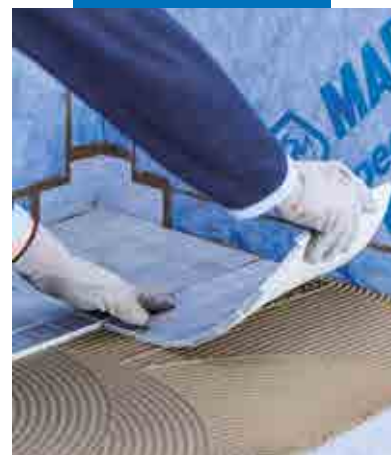
Laying of the tiles
