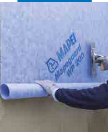
Laying Mapeguard WP 200
