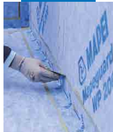
Application of Mapeguard ST
