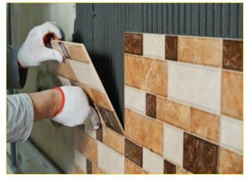
High performance cementitious adhesive with no vertical slip and extended open time for ceramic tiles. Classified as C2TE according to ISO 13007-1 and EN12004
