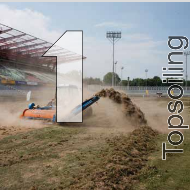
Topsoiling of the old natural grass surface
