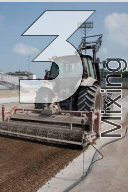
Mapesoil 100 / Mapesoil 50 with a stoneburler
