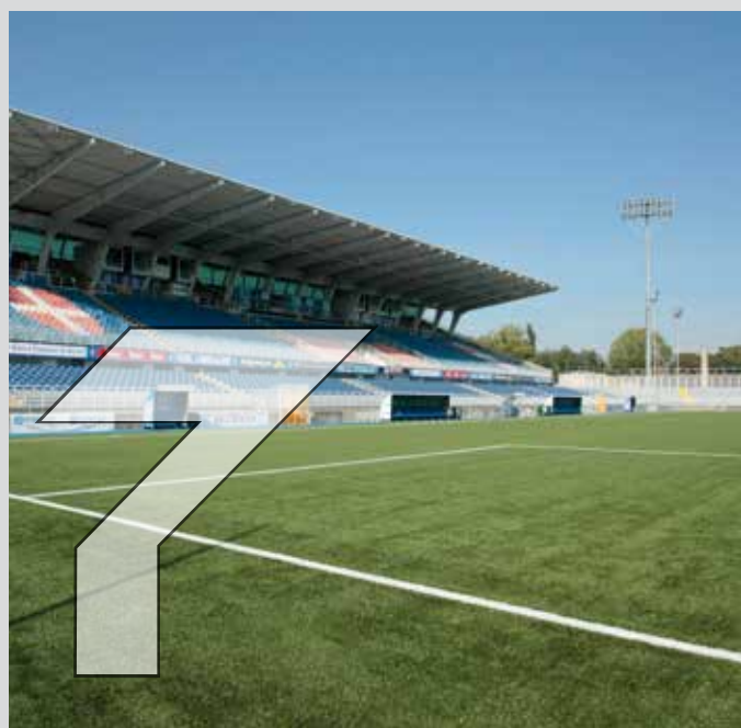
Synthetic grass playing field with horizontal drainage made using Mapesoil 100 / Mapesoil 50
