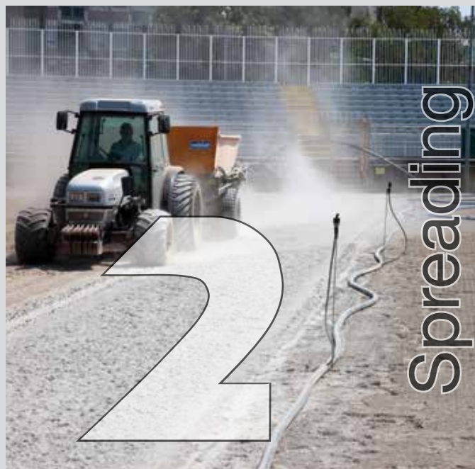
Spreading on the Mapesoil 100 / Mapesoil 50 with a sandblaster
