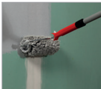
Spreading the first coat of MAPEGUM WPS
