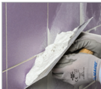
Wall and floor smoothing with PLANIPREP 4 LVT
