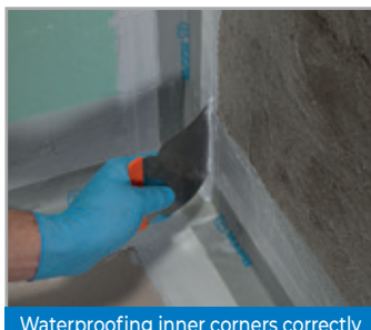
Waterproofing inner corners correctly by applying MAPEBAND PE120 and specially shaped pieces
