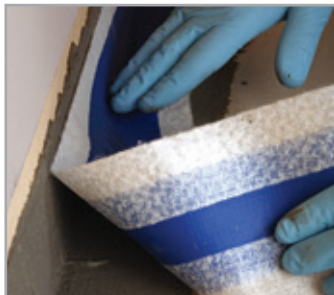
Application of MAPEBAND with MAPELASTIC SMART
