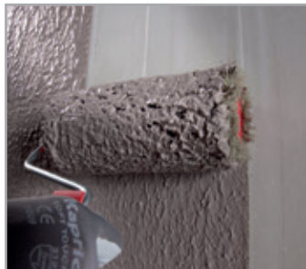
Spreading the first coat of MAPELASTIC SMART with a roller
