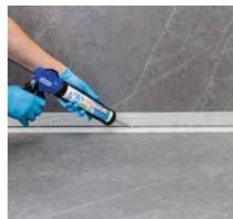
According to current standards, apart from respecting the position of structural joints, control joints and expansion joints must also be included. When installing tiles or slabs **on internal surfaces**, perimeter deformation joints and control joints must be created **every 24-25 m**<sup>2</sup> for ceramics and **every 20-25 m**<sup>2</sup> for stone.
