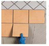
Apply the desired thickness of Kerabond T using the suitable notched trowel depending on the type and size of tile.
