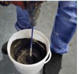
Pour 25 kg bag of Kerabond T into the bucket and mix to obtain an homogenous paste. Leave to rest approx. 5 minutes and remix.
