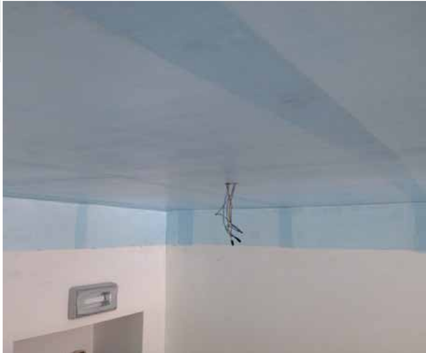
1 | Anti-collapse system for ceilings using the MapeWrap EQ System "Mother Teresa of Calcutta" Comprehensive School - Toro (Campobasso)
