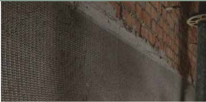
4 | Shear strengthening of bay walls with Mapegrid G220 and Planitop HDM Maxi Sant'Agostino Primary School - Ascoli Piceno
