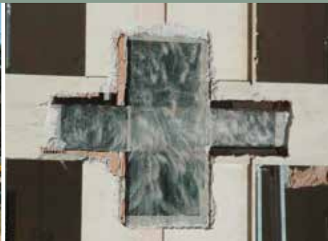
4 | Shear strengthening of bay walls with Mapegrid G220 and Planitop HDM Maxi Sant'Agostino Primary School - Ascoli Piceno
