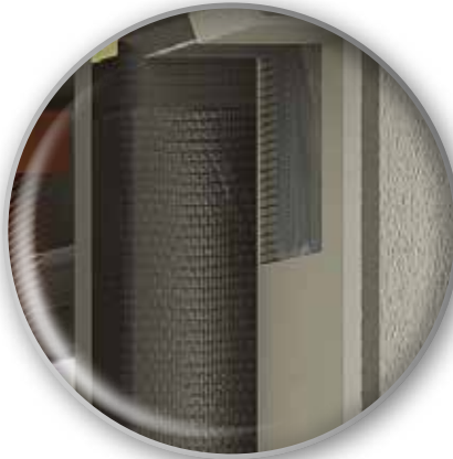
External connections between buffer walls and the reinforced concrete structure (anti-tilting system) using mesh and mortar from the FRG System line
