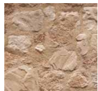
Reconstruction of a stone facing wall
