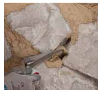
Pointing “exposed” masonry
