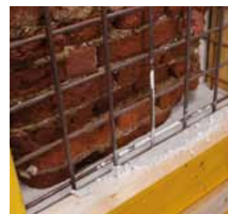
An area of the masonry mortar after pouring
