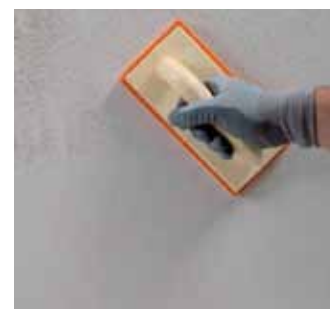
Finishing off the surface with a sponge float
