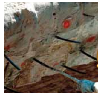
Consolidation of stone masonry
