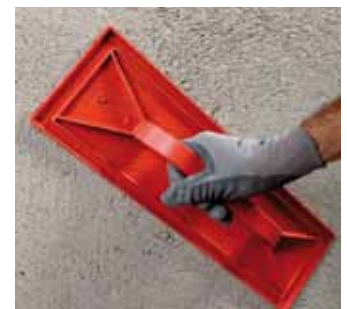
Levelling off the dehumidifying render
