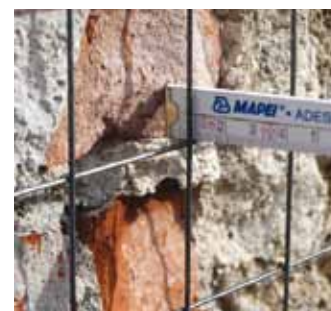
Checking the gap between the mesh and substrate
