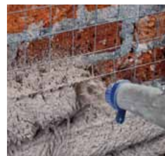
Application of the “structural” render with a rendering machine
