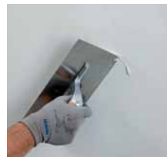
Application of the second layer of ultra-smooth texture skimming mortar
