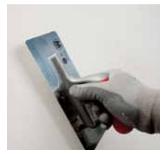
Smoothing over the surface with a flat metal trowel
