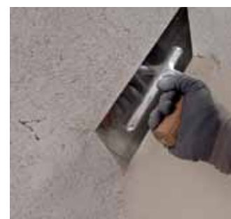
Application of coarse texture skimming mortar
