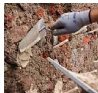
Fastening the small rubber injection tubes in place
