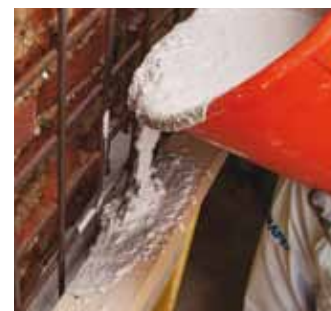
Pouring the mortar made from Mape-Antique Hi-Flow and Gravel 6-10
