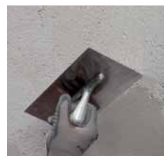
Application of fine texture skimming mortar
