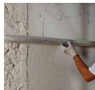
Compacting the dehumidifying render with a straightedge
