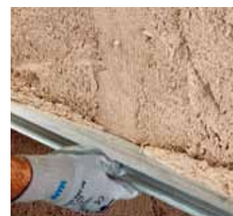
Compacting the dehumidifying render with a straightedge
