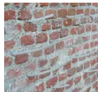
Consolidation of a brick parapet wall
