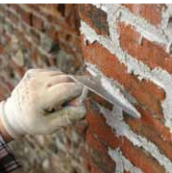
Pointing between brickwork
