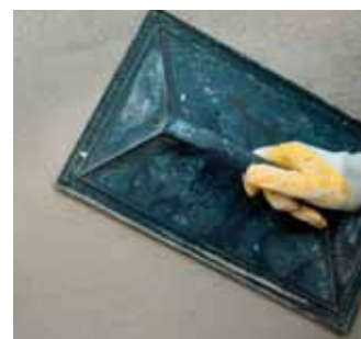
Levelling off the transpirant render
