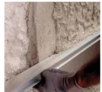
Compacting the dehumidifying render with a straightedge
