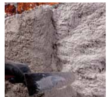
Application of dehumidifying render
