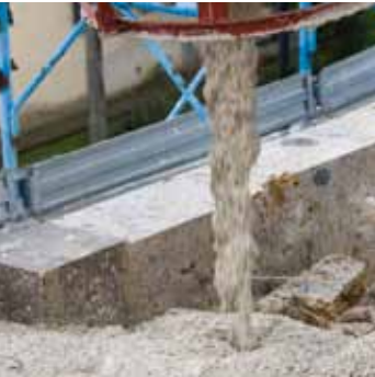
Casting mortar into formwork
