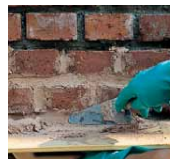
Pointing between brickwork
