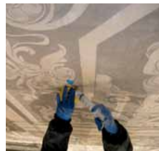
Re-establishing the adhesion of decorated render
