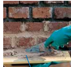
Pointing between brickwork
