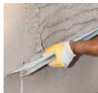
Compacting the transpirant render with a straightedge
