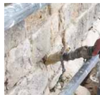
Consolidation of “rubble masonry” stone masonry
