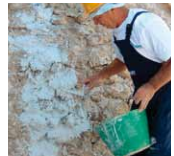
Application of a scratch-coat layer by trowel
