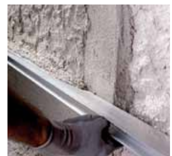
Compacting the dehumidifying render with a straightedge
