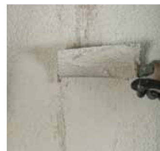
Application of dehumidifying render
