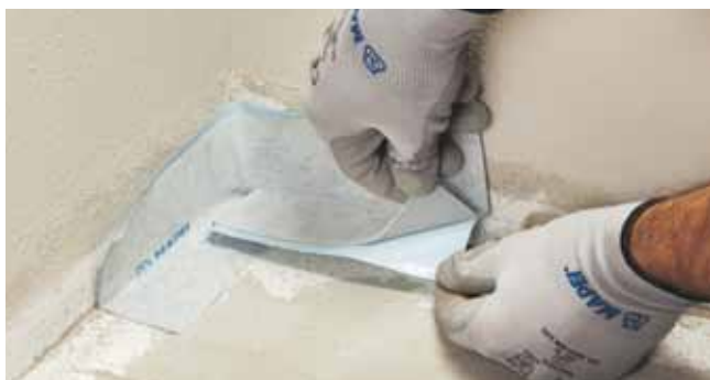
Applying Mapeband SA in corners
