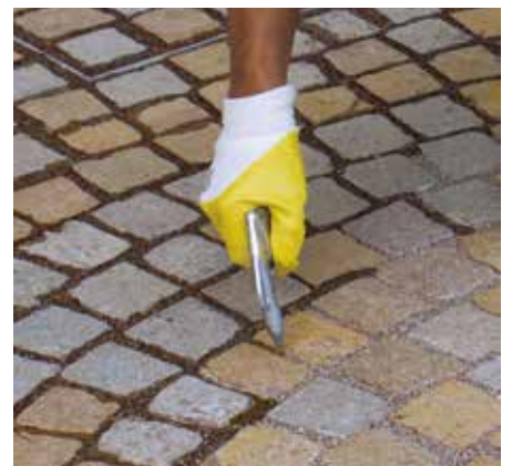
Fill the grouts with Mapestone Joint resin
