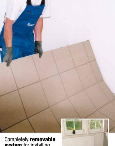
Completely **removable system** for installing ceramic tiles and stone
