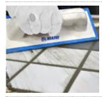
Fill the joints completely, using the Mapei grout float. Remove excess material by moving the float diagonally across the joints.
