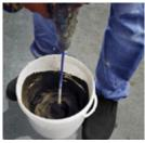
Pour a bag of **Ultracolor Plus** into the bucket and mix to obtain a homogenous paste, leave to rest approx. 2-3 minutes and briefly re-stir before use.
