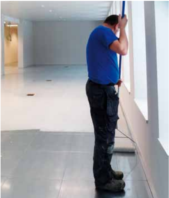
Applying Ultrabond Eco Tack LVT on metal raised floors
