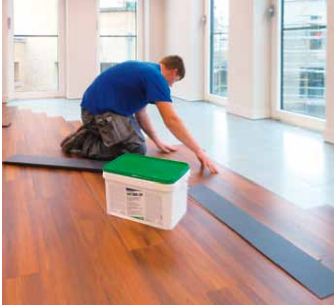
Applying LVT onto a dry film of Ultrabond Tack LVT
