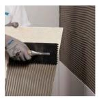
When installing ceramic tiles externally to walls and floors, for large sized tiles and floors subject to heavy loads and for thin porcelain tiles, we recommend that the adhesive is also spread on the backs of the tiles with the suitable notched trowel to ensure there are no gaps to avoid the risk if fracture when in service.
