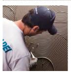
To obtain a good adhesion to the substrate apply a thin coat of **Ultralite** using the smooth side of the trowel. Then immediately apply the desired thickness of **Ultralite** using the suitable notched trowel depending on the type and size of tile.
