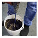
Pour 15 kg bag of **Ultralite** into the bucket and mix to obtain an homogeneous paste. Leave to rest approx. 5 minutes and remix.
