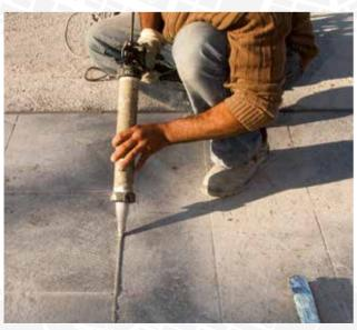
High-modulus, rapid-hardening polyurethane adhesive and sealant for movements of up to 20%. Suitable for sealing external expansion joints. Its high modulus of elasticity means it is suitable for surfaces subjected to intense traffic. Suitable for sealing joints in ceramic floors, including in areas subjected to intense traffic, and surfaces used by vehicles.
