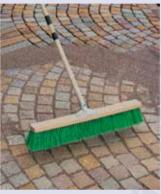
Fill the grout lines with 3/6 mm stone chippings
