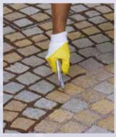
Fill the grout lines with **Mapestone Joint**
