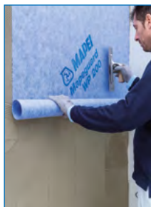
Application de Mapeguard WP 200
