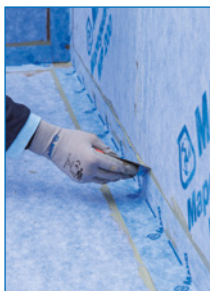
Application de Mapeguard ST
