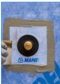
Application de Mapeguard PC
