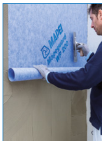
Application de Mapeguard WP 200
