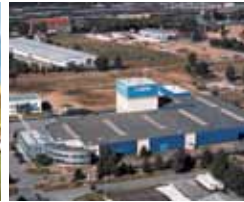
Mapei France S.A. Saint Alban (Toulouse) France
