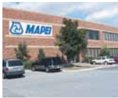
Mapei Inc. Toronto - Ontario - Canada
