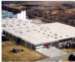
Mapei Corp. West Chicago (IL) - USA
