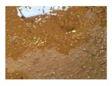
coating along the length of the crack. Tape over the edges of the intervention area. Rout out the crack with a rotary disc, clean the crack walls with a solvent and bevel the edge of the bonded coating alongside the crack. Caulk the joint with a
