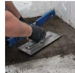
Apply two coats of *Mapelastic®*AquaDefense waterproofing and crack-isolation membrane per instructions outlined in the Technical Data Sheet.
