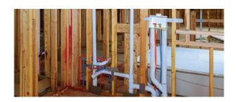
2 Install drain fittings according to building code requirements and build shower base using *Planislope™ RS* polymer-modified sloping mortar.
