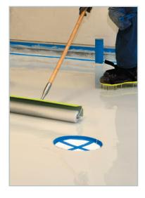
If slip resistance is desired, apply an intermediate coat of *Mapecoat I 24* and broadcast with silica sand #32
