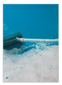
Finish with a coat of Mapecoat I 24 at 9 to 15 mils
