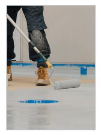
Apply a priming coat such as  $Primer\ SN^{\text{TM}}$  or  $Mapefloor^{\text{TM}}\ I\ 900$  at 9 to 15 mils
