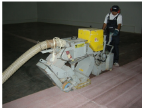
Shot blasting treatment on tiles and old concrete surfaces.
