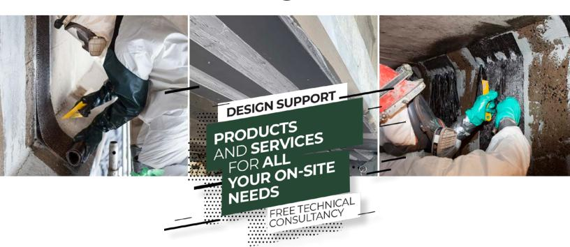
Structural strengthening systems of reinforced concrete, masonry and wooden structures composed of fabrics, pultruded carbon composite plates and rods and epoxy resins.
