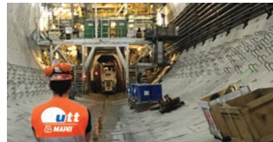
Underground tunneling products
