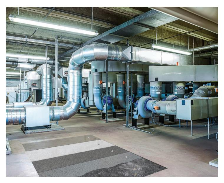
This system is specifically designed to enhance adhesion of multilayer floor systems. It is typically applied on concrete surfaces that require re-profiling or to protect new concrete floors in heavy duty environments. This 100%-solids epoxy resin provides high abrasion and impact resistance, making it an excellent solution for floors subjected to high forklift traffic in which the surface could also be wet.
