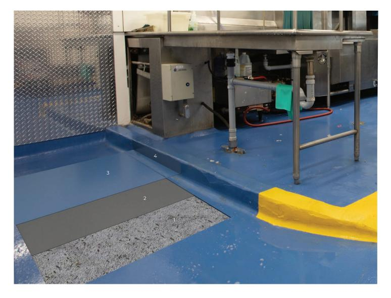
This is the right solution for floors subjected to medium-high loads and/or forklift traffic, high chemical and mechanical stresses, and subject to thermal shock.
