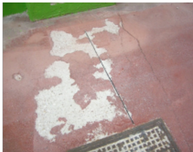
Shotblasting treatment made cracks deeper and wider and removed all loose and friable parts.
